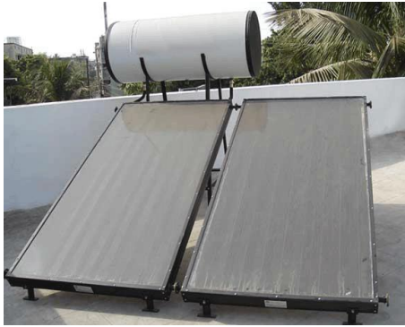
Figure: Solar Water Heater
